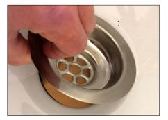
The image above is to help confirm the location of the sealant, the seal is between the top of the ceramic sink and base of the steel "cup".
