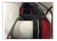
Fit the waste pipe into the opening of the waste disposals body, line up the flange bracket and screw down with the screws/ bolts provided.
